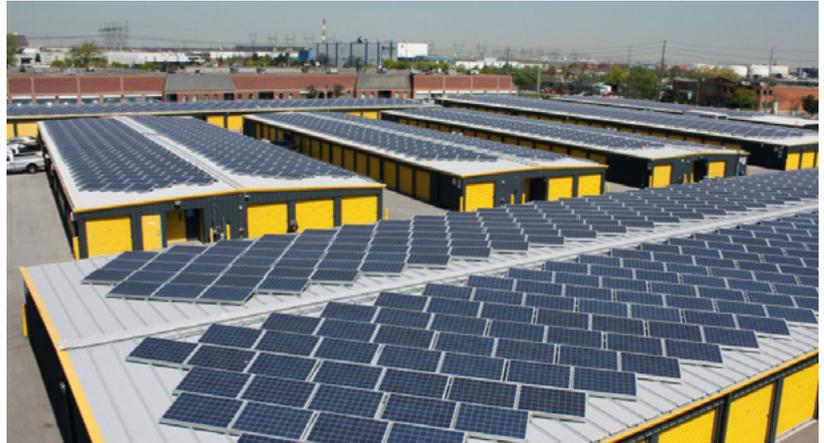
A particular risk for such systems is damage from wind gusts. But if you're trying to design a wind-resilient solar array, you'll hit a wall: Good engineering guidance from traditional sources just doesn't exist.
