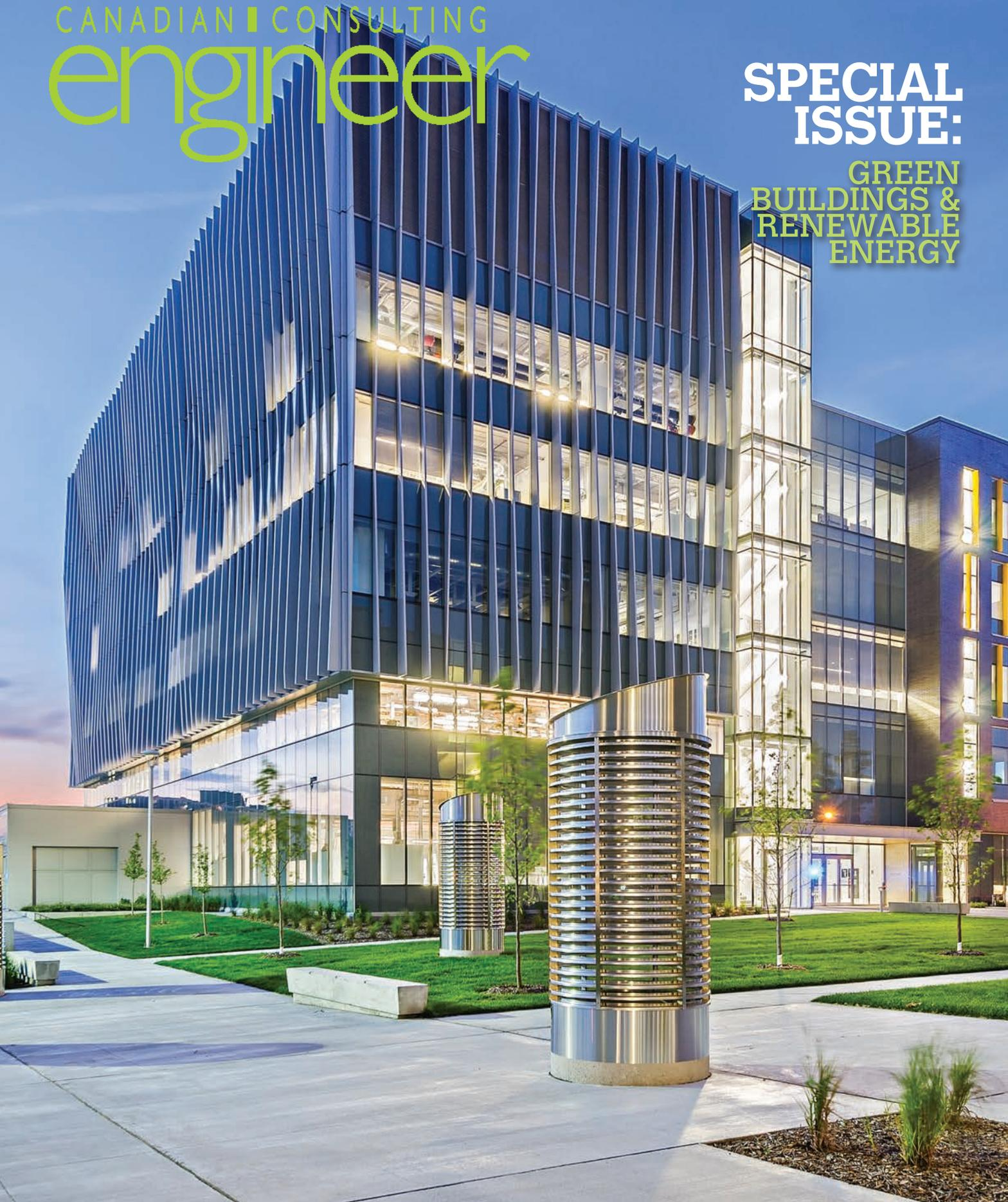
At the Environmental Science and Chemistry Building at University of Toronto Scarborough, massive earth tubes that temper incoming air help to reduce the energy use.
