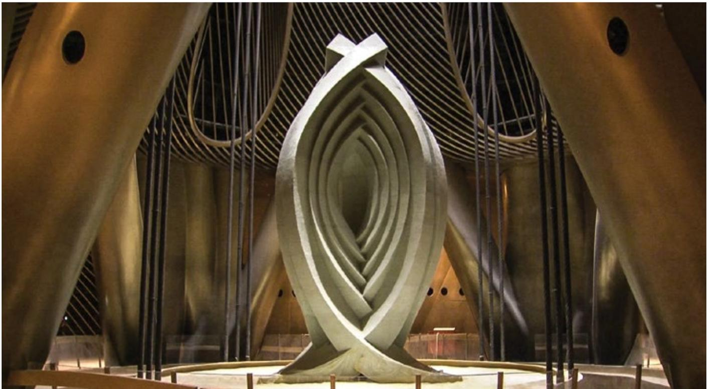
Visitors to the observation area at the top of the Shanghai Tower can see the slow movements of a 70-ton jade sculpture mounted atop the tower's pendulum-like tuned mass damper.
